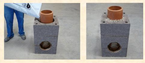
The blocks may be joined together to facilitate the erection of a chimney on an outside elevation attached to a stove, or within the property connected to a traditional fire or modern stove.
